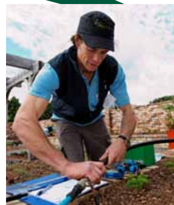
Arboriculture representative Marc Higgie works on the irrigation challenge
